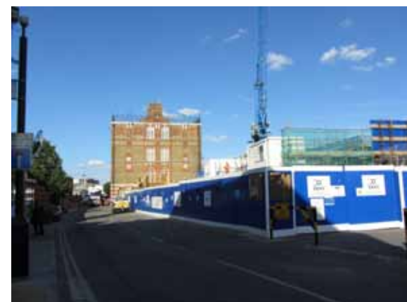
Current view from east along Durward Street
